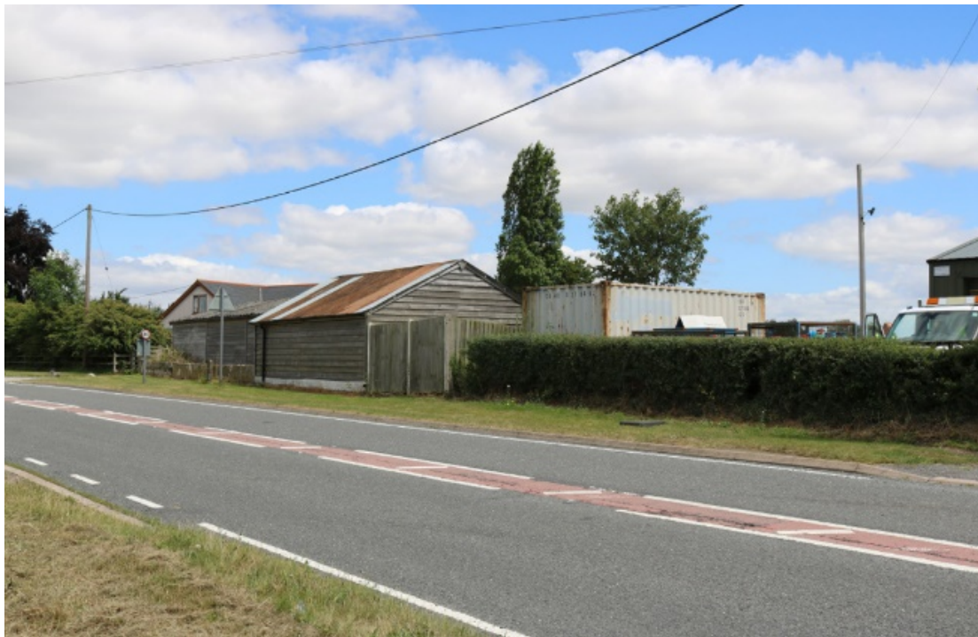
Plate 6: View towards Site 03 from the west on the B1057 showing the stables in the foreground and the existing dwelling beyond, with part of the adjoining depot to the right, behind the hedge
